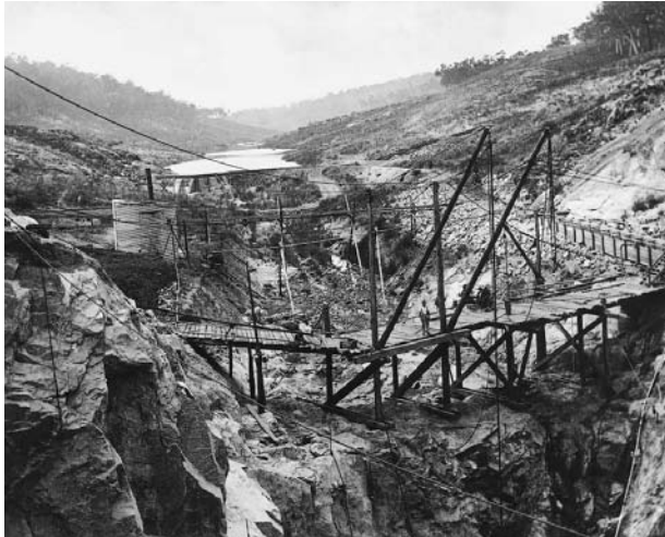
Building the weir wall 1900
