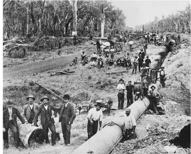
BL 816Bc6844 Pipe-laying across Darling Range c.1900
