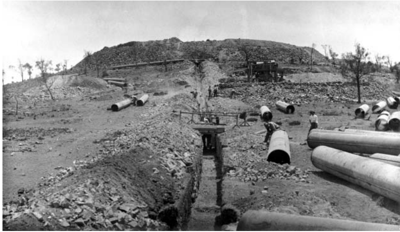
Laying pipe at Mount Charlotte 1902
